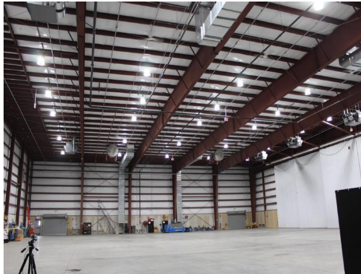
Pilot #1: Quonset Airport Hangar with new PET powered Solid State Lighting
