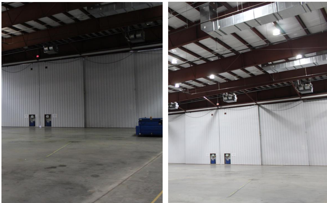
Figure 3-3: Hangar lighting, before (left) and after (right) retrofit
