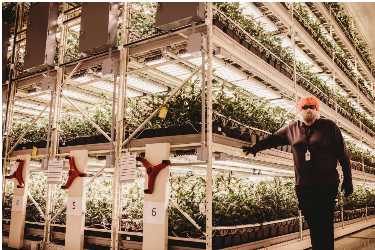
Fig. 4. Following this experiment, Greenseal Cannabis converted their two-level HPS lighted flower rooms to 5 and 6 level high-intensity, LED lighted rooms.
